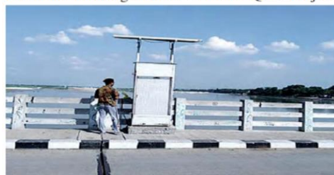
RTWQM station at Shuklaganj, Kanpur (UP26)
