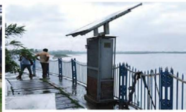
Monitoring station at Barrage at Kanpur (UP19)
